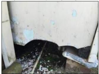
Plate 4 – damaged exterior ACM sheeting at 50 Edmondson Avenue.
