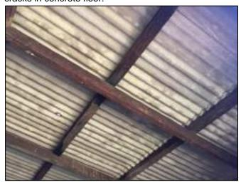
Plate 10 – ACM roofing in shed and attached garage.
